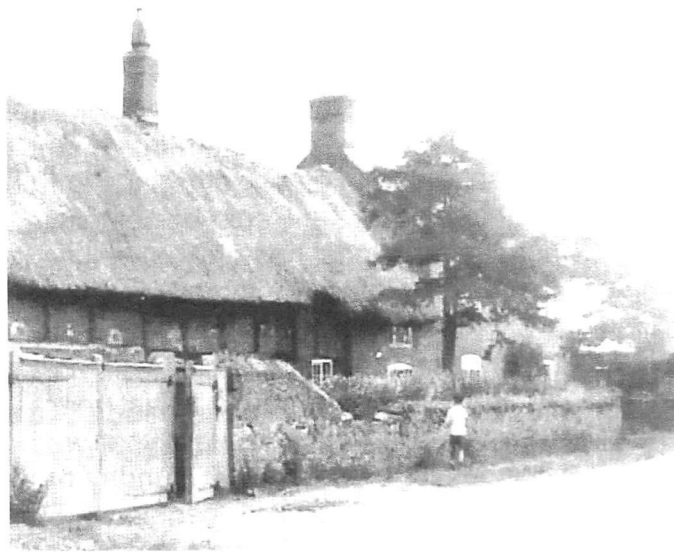
Photo: Church Farm in 1930. Note the box frame structure and thatched roof.
